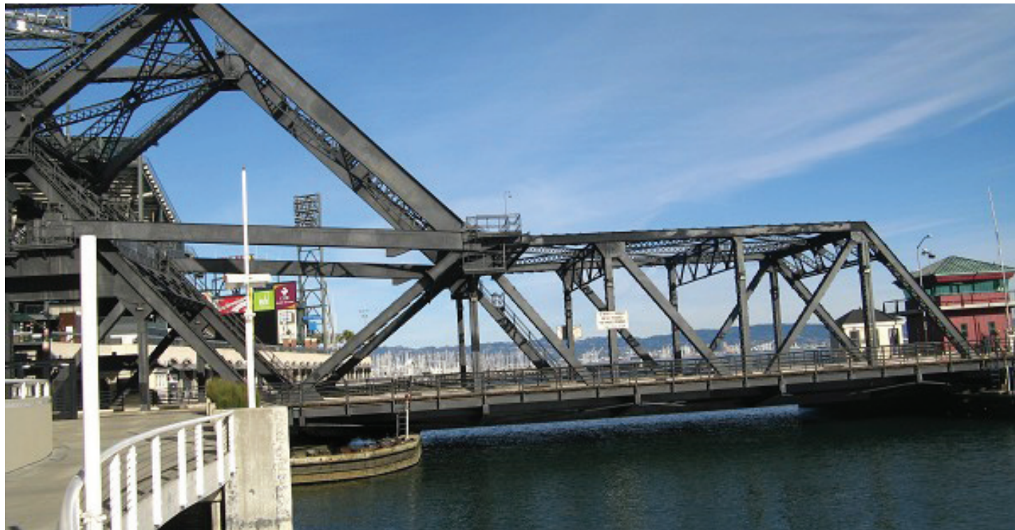
The Lefty O'Doul Bridge (also known as the Third Street Bridge or China Basin Bridge) San Francisco, California
